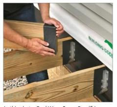
In this photo, DeckWrap PowerBond® is being used on both the ledger board and joist ends where the ACQ wood will come into contact with the metal joist holders.
