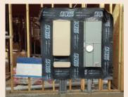
FutureFlash® is an excellent flashing material around vents, electrical boxes and other exterior penetrations.
