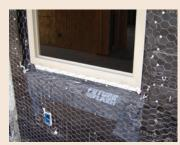
FutureFlash® is ideal to effectively flash complex recessed window assemblies to prevent water damage.
