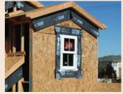
FutureFlash® is designed to create a waterproof and self-sealing envelope in all building applications.
