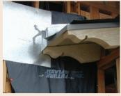
Tough, UV-friendly FutureFlash® prevents leaks at a facia board/wall termination and separates dissimilar metals to prevent corrosion.
