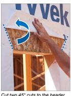
Cut two 45° cuts to the header section and fold up and hold with staples or membrane.
