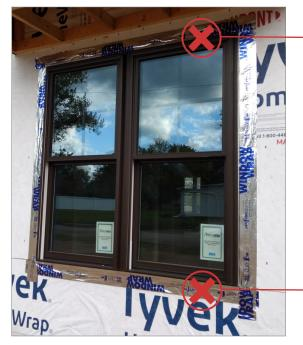
House wrap was wrapped inside the structure. If water penetrates behind the house wrap, it can funnel right into the structure.
