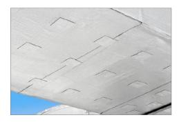
On ducts over 24" (60cm) wide, pin bottom 12" (30cm) on-center. Cover pins with a minimum piece of 3" (7cm) squares of FlexClad<sup>®</sup> to seal pins from weather.
