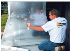
It can also be applied at overlap areas for improved adhesion. Apply a light coat direct to the substrate and wait 2-3 minutes, depending on humidity and wind conditions, or until surface no longer looks wet.
