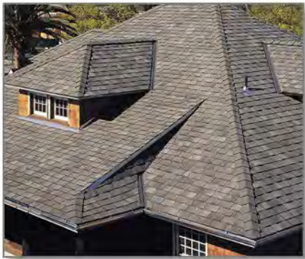
Asphalt Shingles
