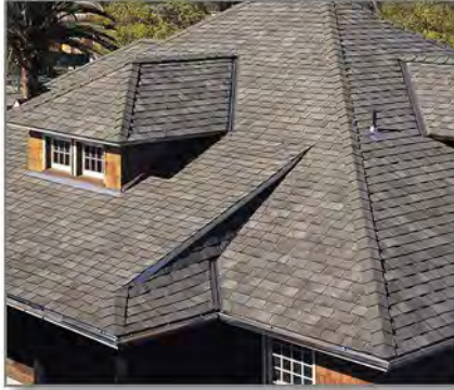
Asphalt Shingles
