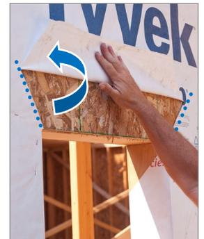
Cut two 45° cuts to the header section and fold up and hold with staples or membrane.
