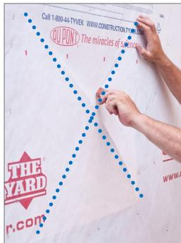
Cut an "X" pattern in the house wrap from corner-to-corner of the rough window opening..
