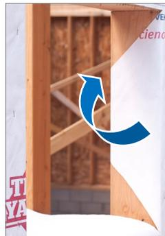
Wrap both jamb sections into the rough window opening and secure tightly with staples.
