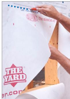
Cut the header section flush with the top of the rough opening and discard.
